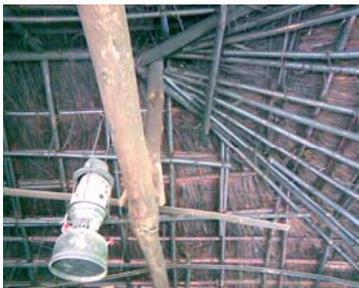
Fig. 28. Bamboo beams &thatched roof
