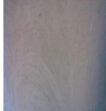
Fig. 21 .Floor cladding with Dung & Husk
