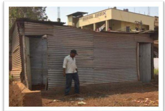
Picture 14: Temporary shed near the Karez
