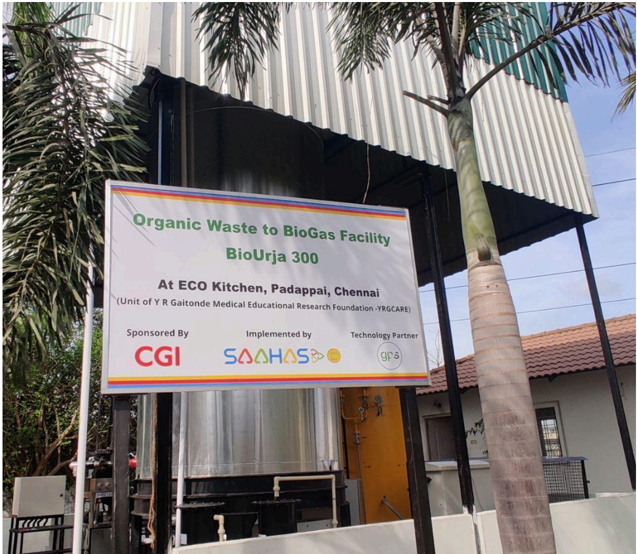
Image 3: Biogas facility at ECO Kitchen, Chennai.
