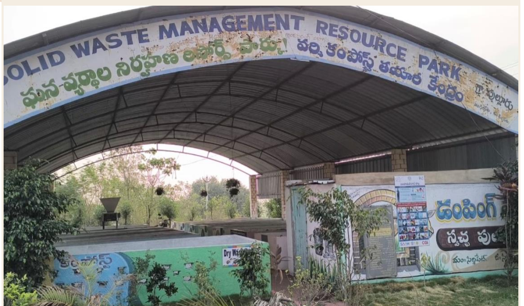
Figure 4: Resource recovery centre at Pullur.
